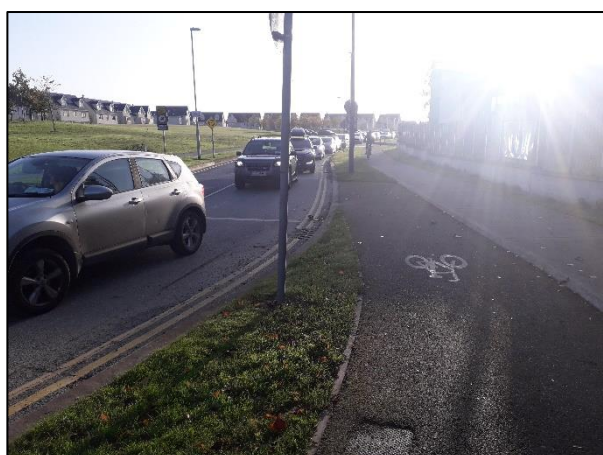
Figure 3.25 Queuing along the access road from the Kilcullen Road signalled junction
