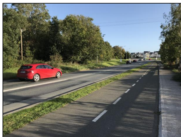
Figure 3.24 Existing Pedestrian and Cycle Facilities on Kilcullen Road
