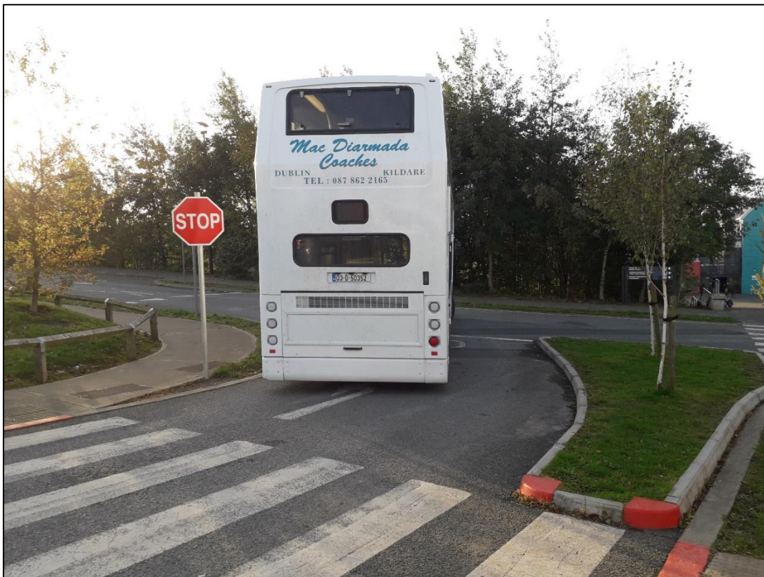
Figure 2.6 Build-out installed in order to prevent traffic from turning right onto the main access road towards St. David’s N.S. and Piper’s Hill College.
